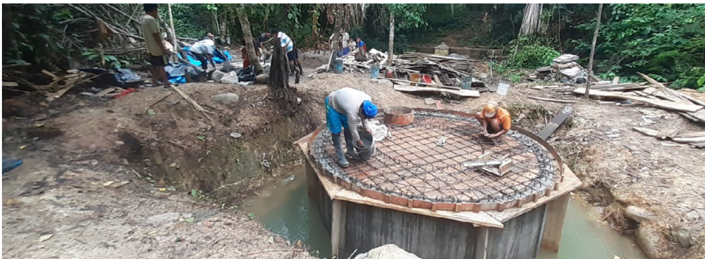
Shenontiari: above: Attaching the rebar before casting the concrete top to finish off the well. below: Community planning meeting for the new water project. This project was completed in 2021.
